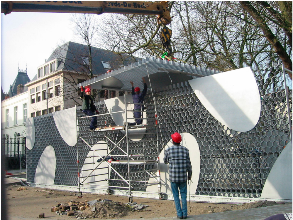
Figure 13. Prefabricated panels were slipped into place on site (© Toyo Ito & Associates ).
