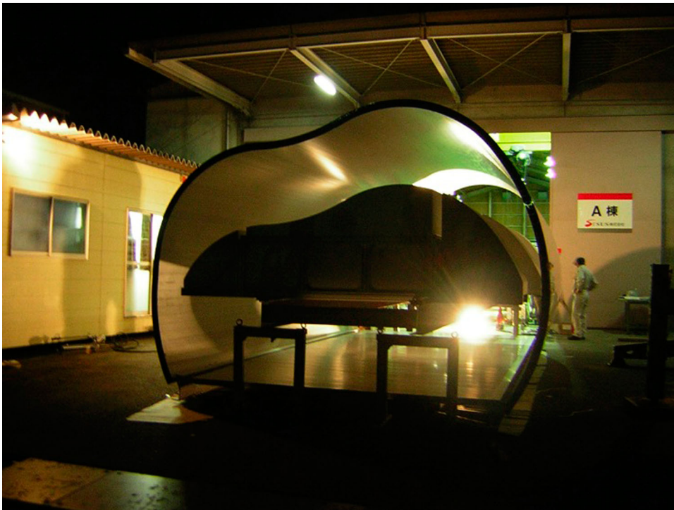
Figure 23. Aluminium container, with plank size evident (© Masato Araya, Oak Structure Design Office).
