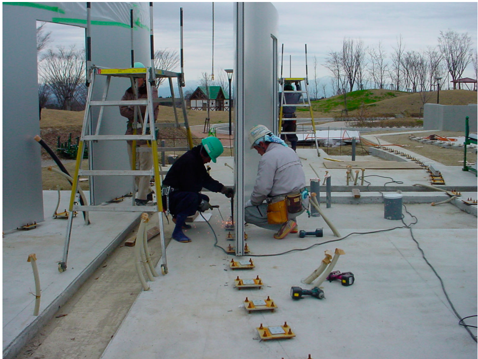
Figure 15. Setting the slim walls (© Toyo Ito & Associates).
