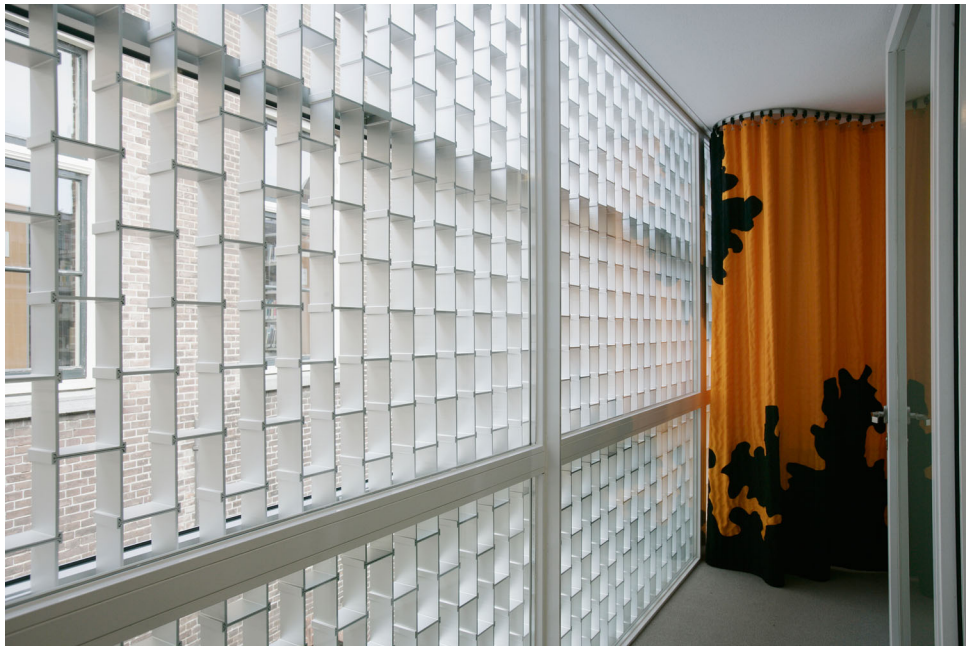
Figure 24. Aluminium brick façade (© Wim te Brake).
